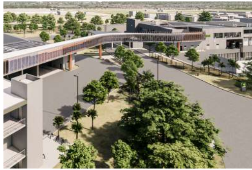
SOUTH DADE TRANSIT OPERATIONS CENTER
