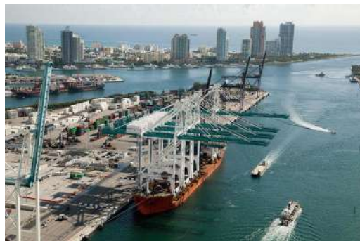
PORTMIAMI WHARVES STRENGTHENING PROGRAM
